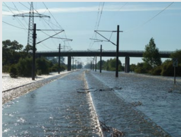
Photo 2.3 Flooding of the Hannover-Berlin railway line
