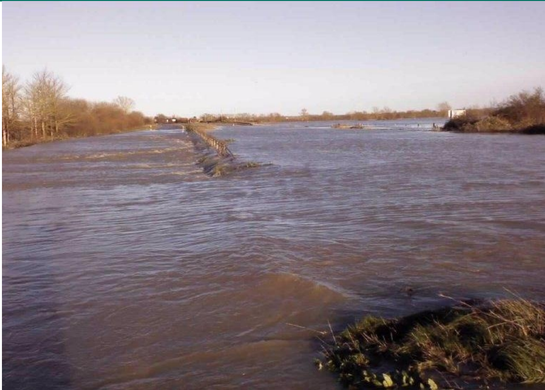
Figure 4.4 - Flooding on the A303 near Ilchester, Somerset
