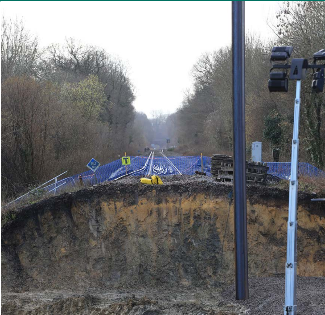
Figure 6.4 - Work underway to repair the landslip at Botley, Hampshire
