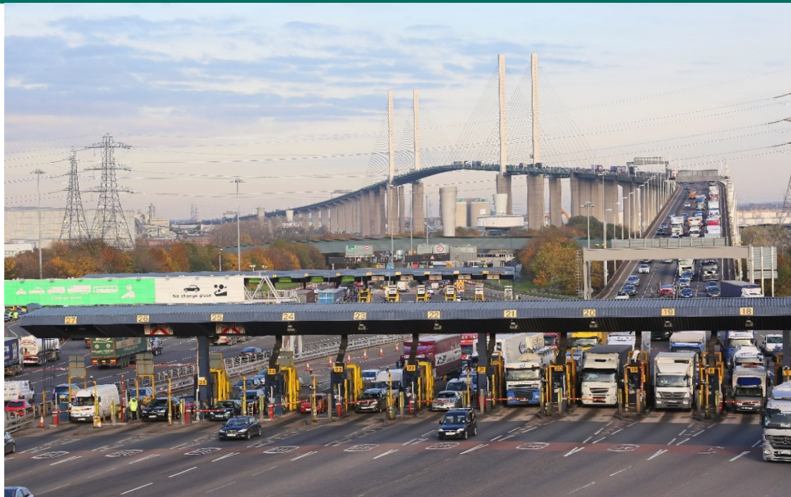
Figure 4.2 - QEII Bridge, Dartford
