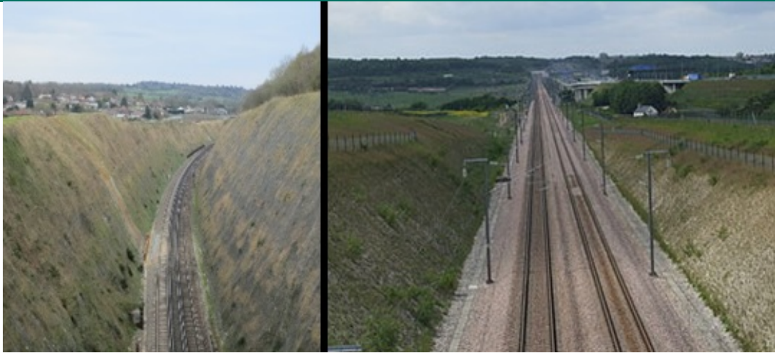
A steep historical cutting shown side by side with the modern design standards used on HS1
