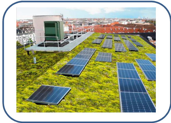
Standard sedum-mos m. solceller
