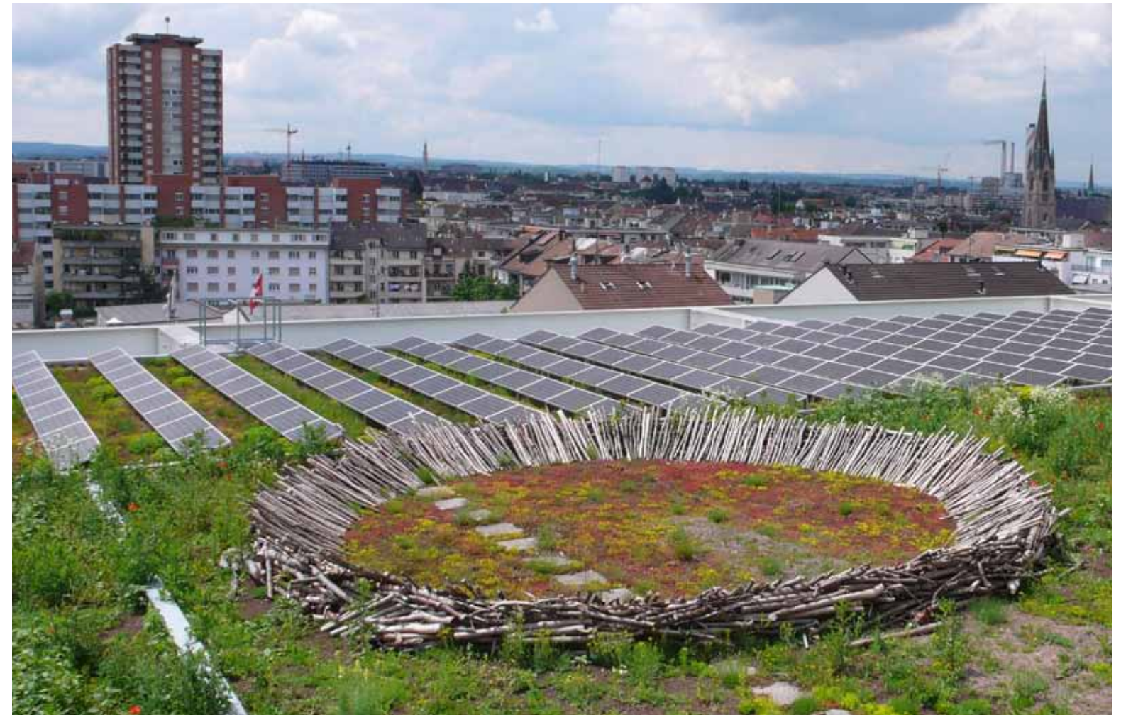
Green roof on the exhibition hall in Basel. The green roof is designed to support biodiversity
